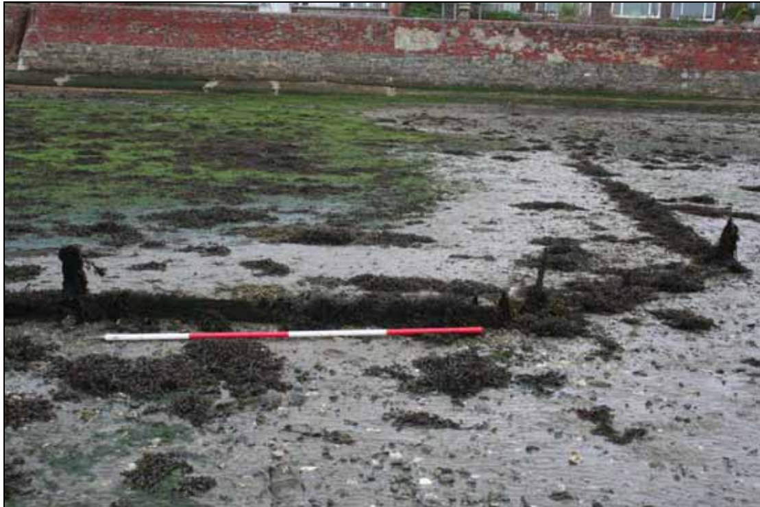
Figure 24: Pit I viewed from the south, showing missing structure on its northern side and the possible sluice structure at its south east corner.
